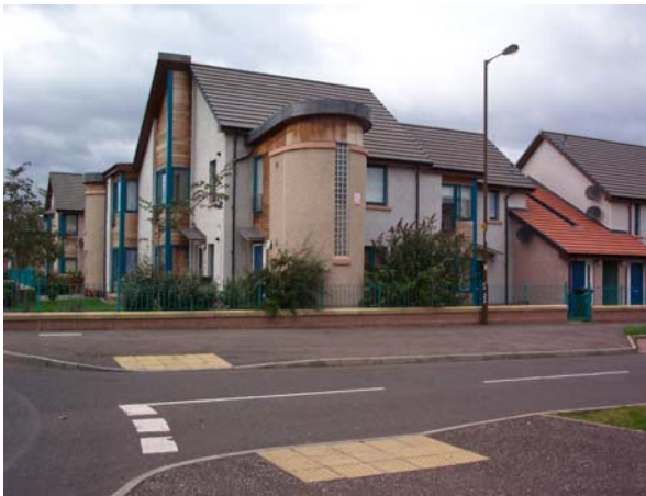
Fig. 6: New Housing Development
